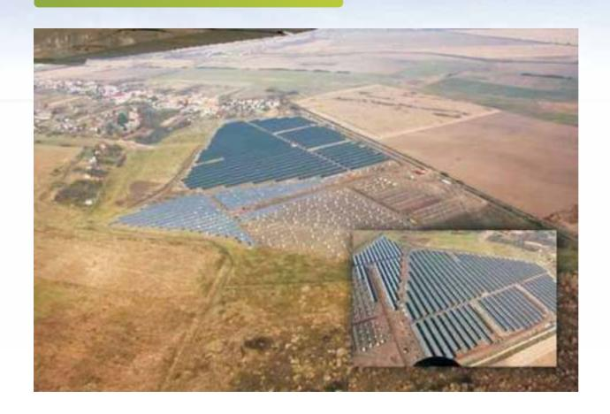
3x 1 MWp FIX 9 Panel polycrystal SUNTECH 280W
