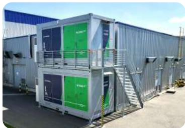
Hanon Systems 864 kWh 970 kWp (FVE)
